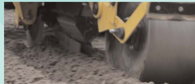
During laying and digging operations
