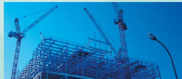
In civil works
